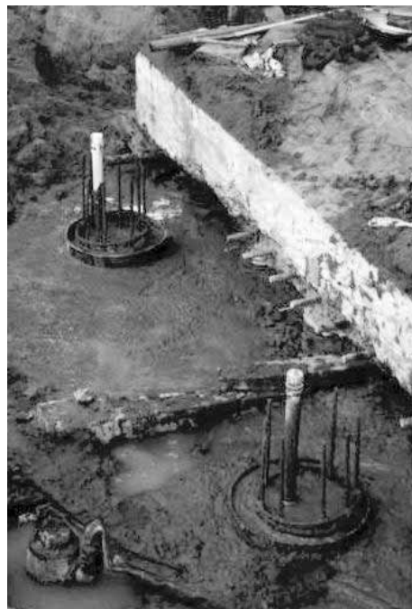
Clean concrete placement with minimum concrete wastage.
