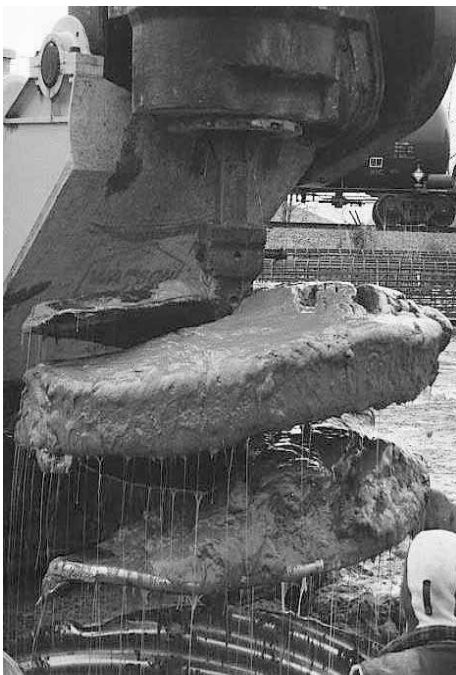
The slurry binds the soil together making excavating easy.
