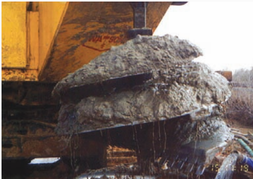
Super Mud binds the soil together making excavating easy.
